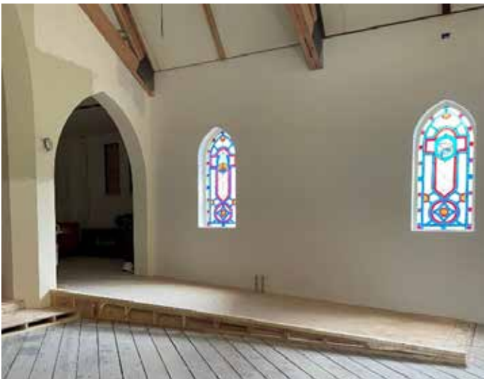
Accessible Ramp ready for Wood Flooring
