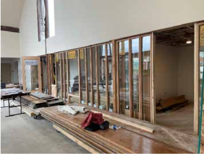
Narthex / Admin Storefront System (Open areas will be filled with reclaimed pew wood and intermittent glass panels will receive an opaque film)
