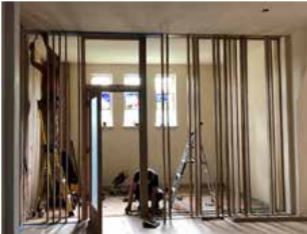
Chapel West Wall (opaque glass is still to be installed)
