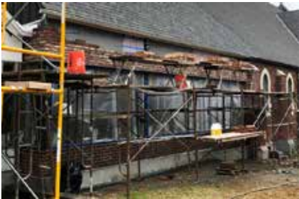
Exterior brick and parge coating.
