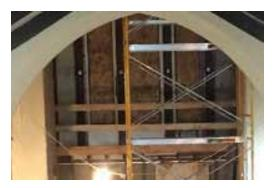
*March 3, 2021* – The structural steel column work for seismic improvements is complete. The last four columns were installed adjacent to and between the tall stained-glass windows on the east end of the Sanctuary. While the process was a little slower than anticipated, everything fit, is secure, inspected, and approved.
