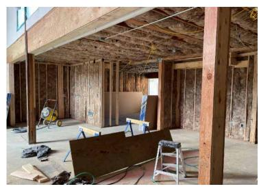
removal of the structure is planned for mid-April and will include the lower-level basement room. The new foundation walls and water proofing is in place to allow backfill of the area immediately following removal.
