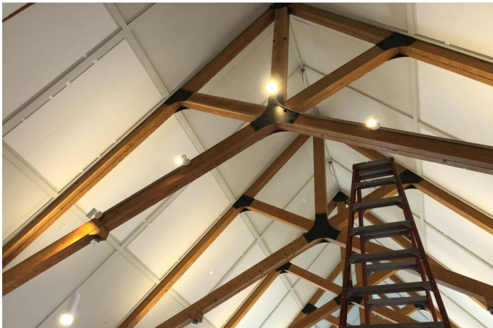
Acoustical panel install underway in the Sanctuary
