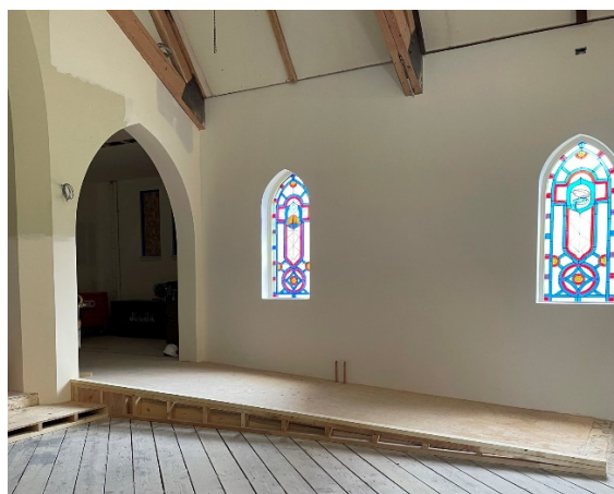
Accessible Ramp ready for Wood Flooring
