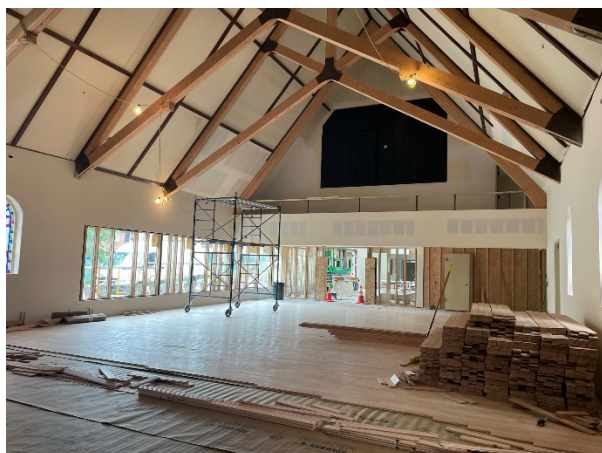
Sanded Trusses, Full Storefront Systems, Wood Flooring
