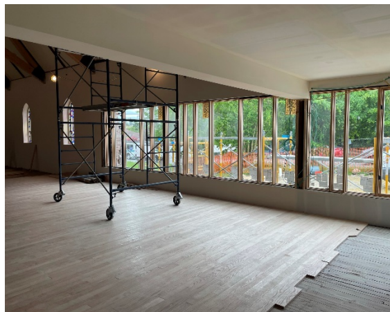
Sanctuary South Wall
