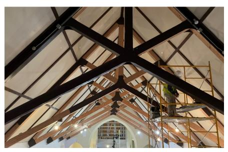
Inside the building, subcontractors are tapping, mudding, and texturing the new sheetrock walls. Trusses in the Sanctuary are being stripped of the dark stain and painting in the lower level and administration will begin in April. Cabinets, ceilings, and lighting will start in May.
