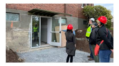
The lower-level entry door, sidelight, and awning have been installed. A concrete entry walk will be placed over the gravel you see in the photo and the full wall will be parge coated (thin layer of concrete) to create a uniform appearance. This is a unique element of the project. The lower portion of the wall was below grade for many years. From inside the building, it is amazing to see how this new entry brings in light and creates a connection to the outside.
