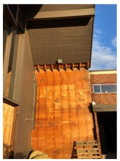
The SW stair tower and Library portion of the building are scheduled for demolition in April. A new beam will be installed at the bottom of this overhand (shown in the photo to the right) to carry the load of the east roof trusses. Once these portions of the building have been removed, restoration of the brick façade and installation of the new window system that spans from the Narthex into the Sanctuary can get underway.
