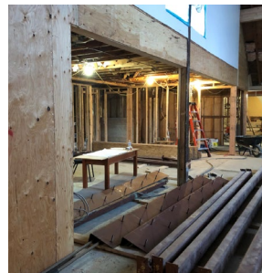
Plywood shear walls at Chancel, Administration, and new Small Meeting Room
