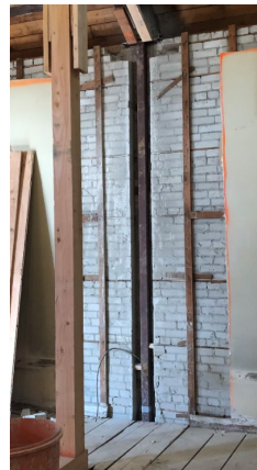
Column Installed
