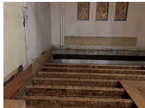
Lowered Chapel Floor Joists
