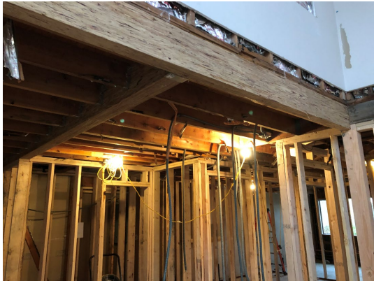
New beam at Narthex and framing in Admin Offices
