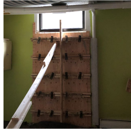
Infill forms at south exterior stair
