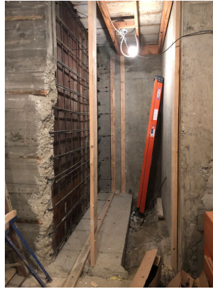
Exterior wall forms at old stair
