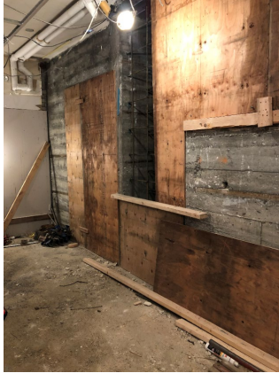
Fireside Room - concrete forms
