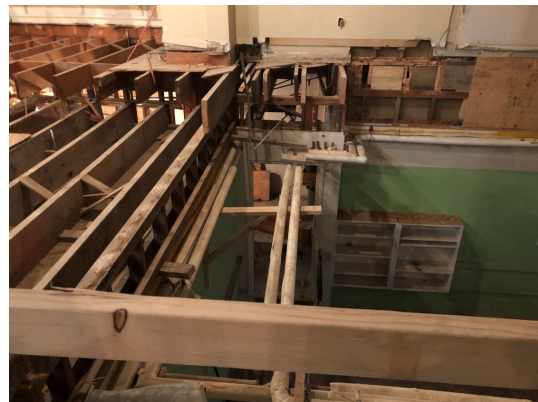
Chapel floor framing removed (to lower) and classroom below
