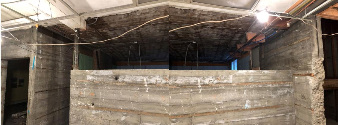
*Fireside Room walls stripped of framing and ready for concrete forms to create what will be exterior, below grade walls after the demolition in the spring.*
