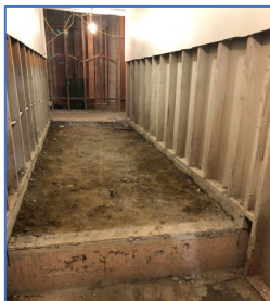
demolition for ramp
