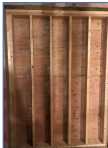
cutout for new exterior door
