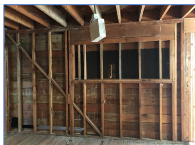
south wall of sanctuary
