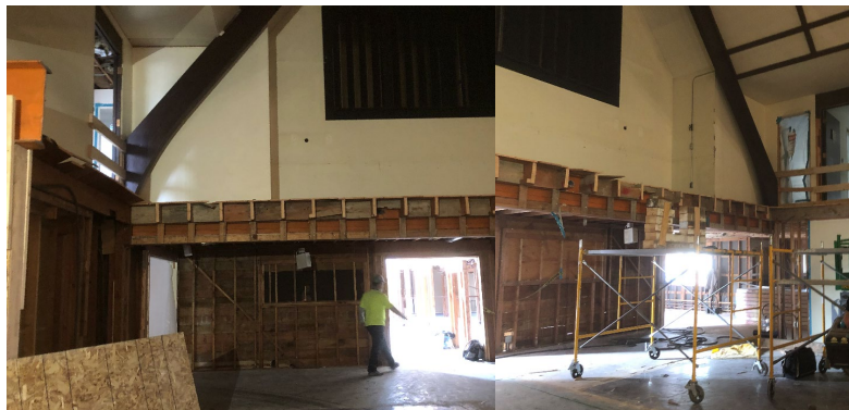
Two photos showing sanctuary/narthex common wall and balcony removed
