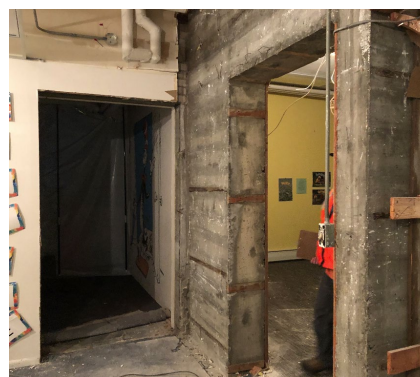
Lower level library structure walls exposed
