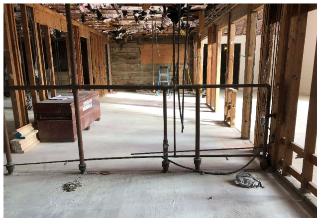
Administration area looking east
